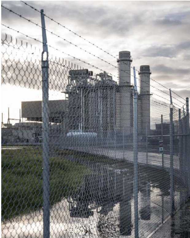
Sutter Energy Center, now closed, made money only if Calpine Corp. found customers for the plant's power. Other large, natural gas plants in the state also face early closures. (David Butow / For The Times)
